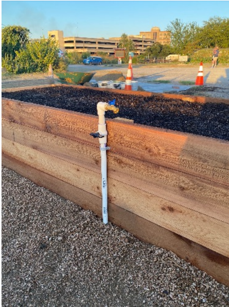
New plumbing at the raised beds. Photo by Jim Willmann
